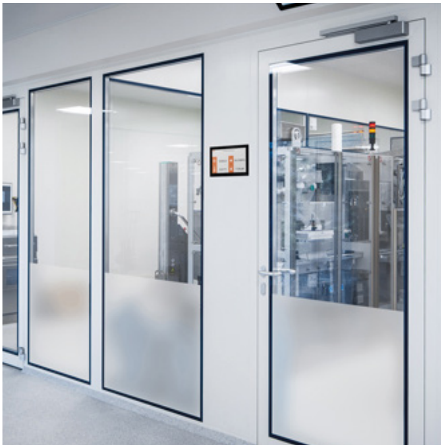
Figure 8: An HMI with a usually small display and limited computing power is used for the user interface of building automation systems.
