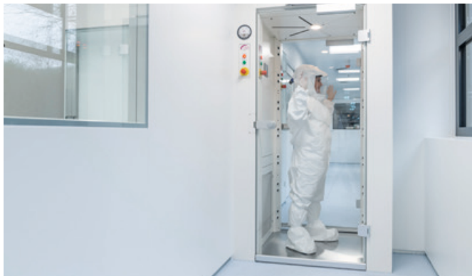
The air shower provides a safe working environment when handling highly potent substances. (Photo: Helmar Lünig, shutterstock.com/Haywiremedia, Harro Höfliger, Andreas Dalferth, Jan Seidl)
