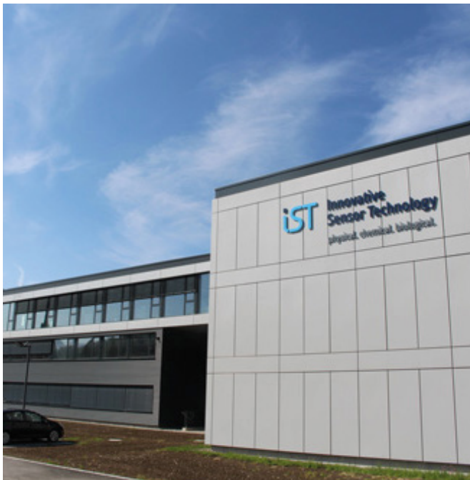
On a path to growth: Innovative Sensor Technology IST AG – a subsidiary of the Endress+Hauser Group – expanded its facility in Ebnat-Kappel at a cost of around 15 million euros.
