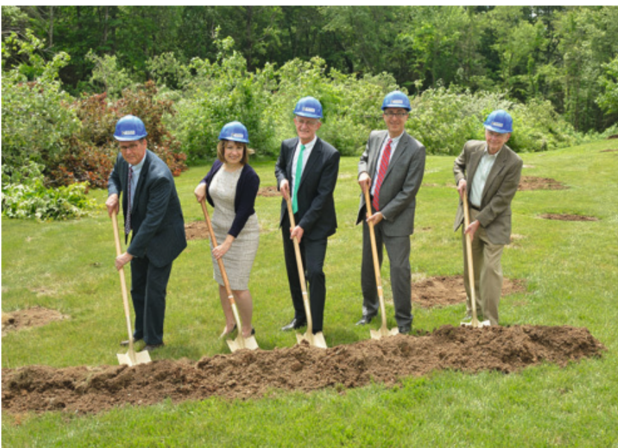
Ground-breaking ceremony for the extension at Arburg's US subsidiary in Rocky Hill (from left): Jim Becker, Project Architect Tecton Architects, Claude-Helene McIntyre, CFO Arburg Inc., Friedrich Kanz, CEO Arburg Inc, William O'Sullivan, Deputy Mayor of Rocky Hill and Larrye deBaer, Chairman of the Economic Development Commission, Rocky Hill. (Photo: Arburg)
