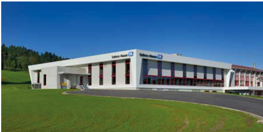
Endress+Hauser dedicated a new production facility in Nesselwang, Germany, after investing more than 10 million euros in the expansion.
