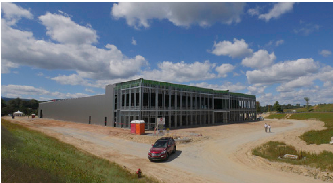
The new facility is taking shape.
